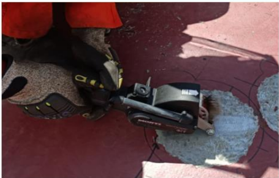
Coating removal & surface roughening with Bristle Blaster or Grit Blasting 005_PT_M_008 [2]
